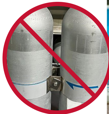
Figure 1: Double bottles with a single band. Two bands are required for the Thermo and XS Isolation manifolds. (U.S. Navy photo by Naval Safety Command)
